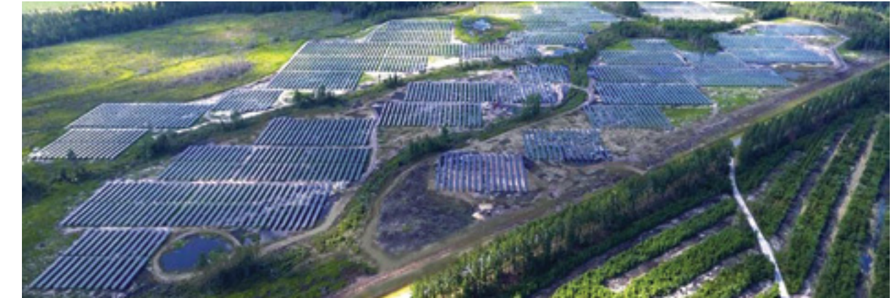
Through strategic investments, we are working to integrate solar projects on rooftops and brownfields, like this one, whenever possible.
